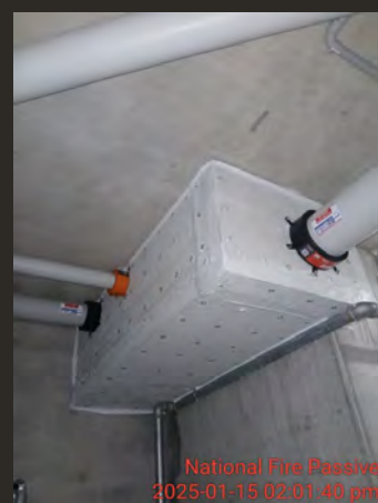
Retrofit fire rated enclosure
