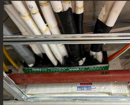
Retrofit Fire Box Installation
